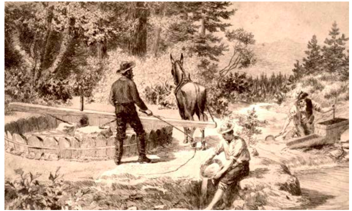
Before the steam-driven stamp mill, there was the arrastra, with a heavy stone dragged around the inside circle to crush ore.
