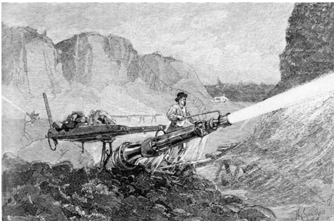
With a load of rocks as counterweight, one miner could control the “prodigious” jet from a hydraulic mining nozzle. From Century Illustrated magazine (January 1883) via Wikipedia.
